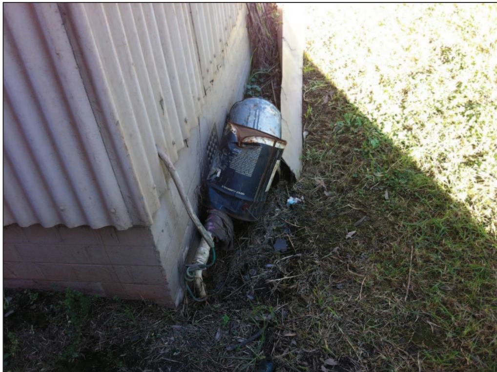
Plate 14 – Empty paint tins adjacent to the western corner of the Coils Factory.
