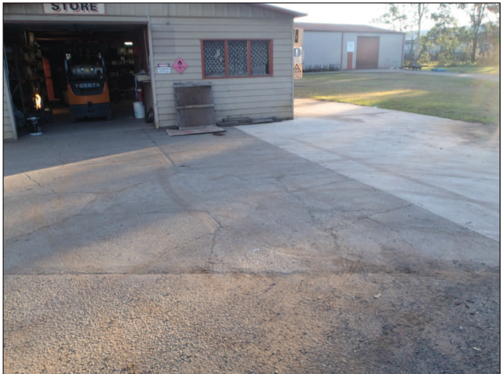
Plate 21 – The area of the decommissioned UST (UST 1) with a store shed (Location 24) beyond.
