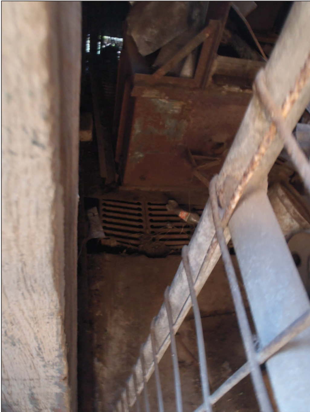
Plate 24 – Drain in Location 28 adjacent to the western wall.
