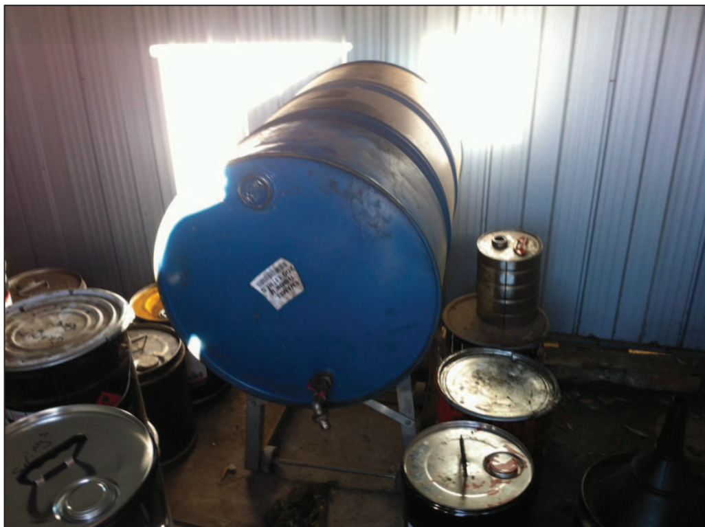
Plate 7 – 200L paint thinner AST (AST 1) inside the flammables shed.
